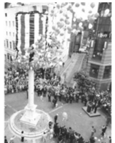
Top: The repaving of Seven Dials, 1986. Camden Council, with Government support completely repaved the circus and created a new island for the Pillar's reconstruction
